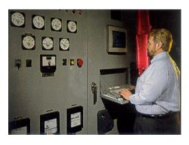
Cogeneration's ability to produce both electricity and steam form natural gas proved a perfect fit for Ajax's operation. Ajax now receives about 35% of their electricity from their own on site generator, and 90% of their steam (recovered from the waste heat off the engine and exhaust) which is used to heat the process tanks that are vital to their finishing and plating precesses. Cogeneration is saving Ajax approximately \$9,000 each month their investment in cogeneration will be fully
